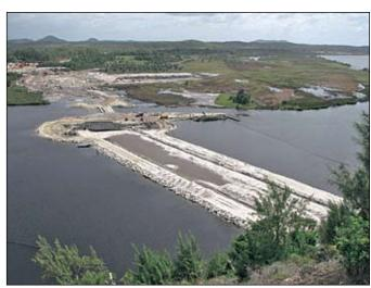
in late 2008. The weir project was initiated to prevent sea water flowing back up the Anony River into Lake Ambayarano, the main water source for the mining operation.
