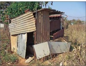
sanitation and hygiene practices. While most of the households surveyed had toilets, many of these were self-built pit latrines in very poor condition, with some in near state of collapse.
