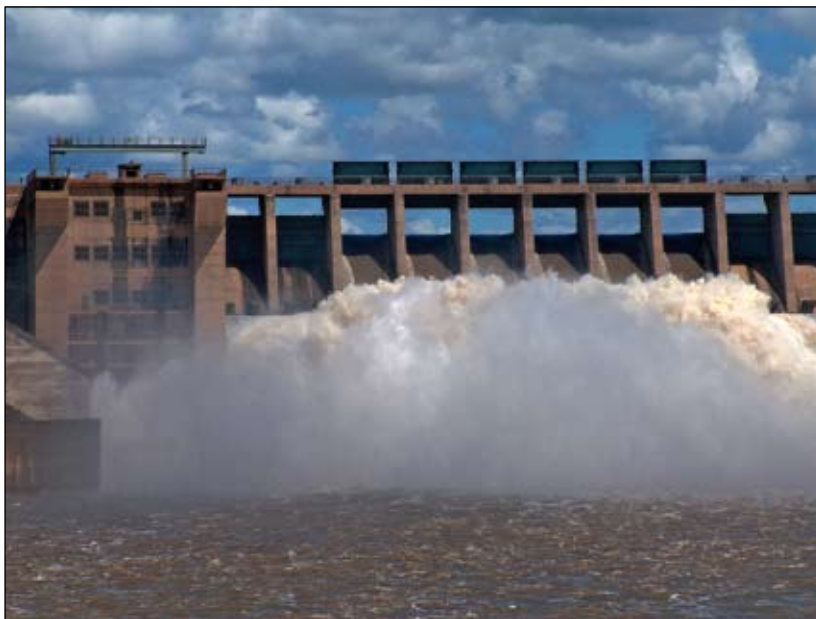
The Vaal Dam has 60 crest gates, each capable of releasing 115 m 3 /s.
