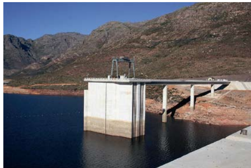
The Berg River Dam intake tower is divided into two sections. The north section is a dry shaft (well) equipped with multi-level inlets, pipes and valves, which provides the facility for drawing water into the Cape Town supply system and provides for low flow environmental releases.
