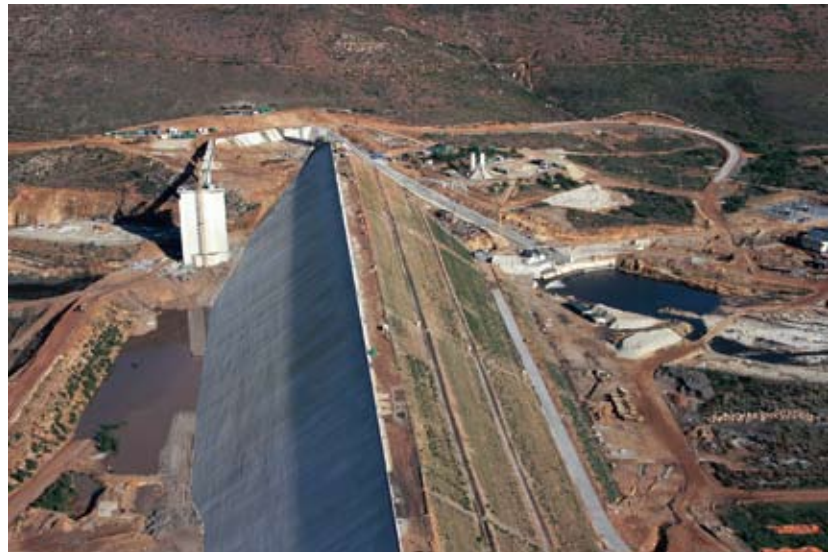
The Berg River Dam is a concrete-face-rockfill dam type. The dam is 65 m high, 990 m wide and 220 m in width. The gross storage capacity of the dam is 130 million m 3 . The outlet works have been designed to release both low flows and high flows with provision for a peak release of up to 200 m 3 /s. This makes it the first dam in South Africa in which provision is made for flood releases for environmental purposes.
