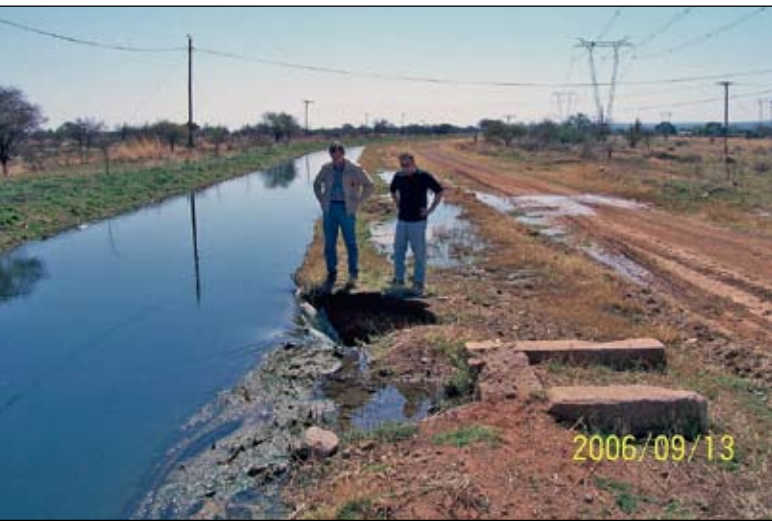
Water loss and structural damage due to flooding can occur as a result of aquatic weeds in irrigation canals.
