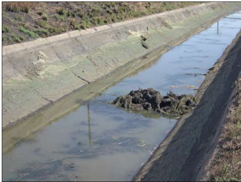
Aquatic weeds are choking many of South Africa's irrigation canals severely affecting performance and water efficiency.
