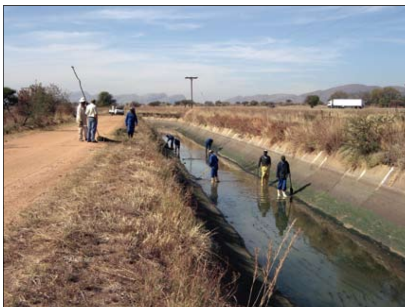
Physical cleanup of aquatic weeds and algae in water conveyance structures is an expensive, labour-intensive process.
