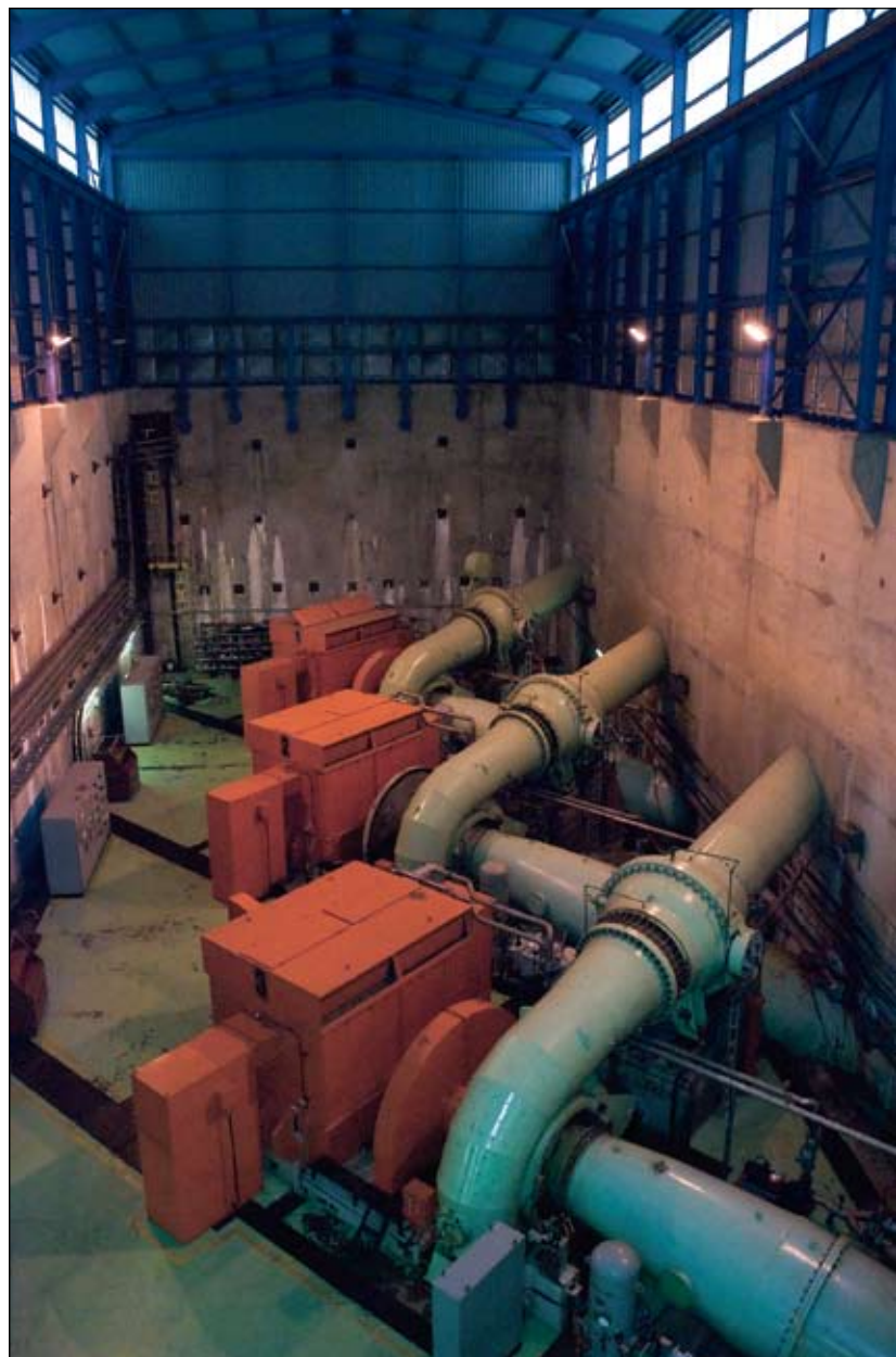
The machine floor at Collywobbles hydroelectric power station, showing the three 14 MW generating units.
