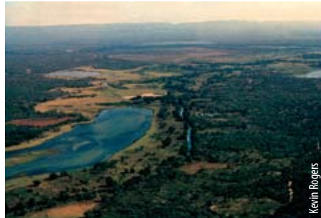
Pongolapoort Dam as seen from the air.
