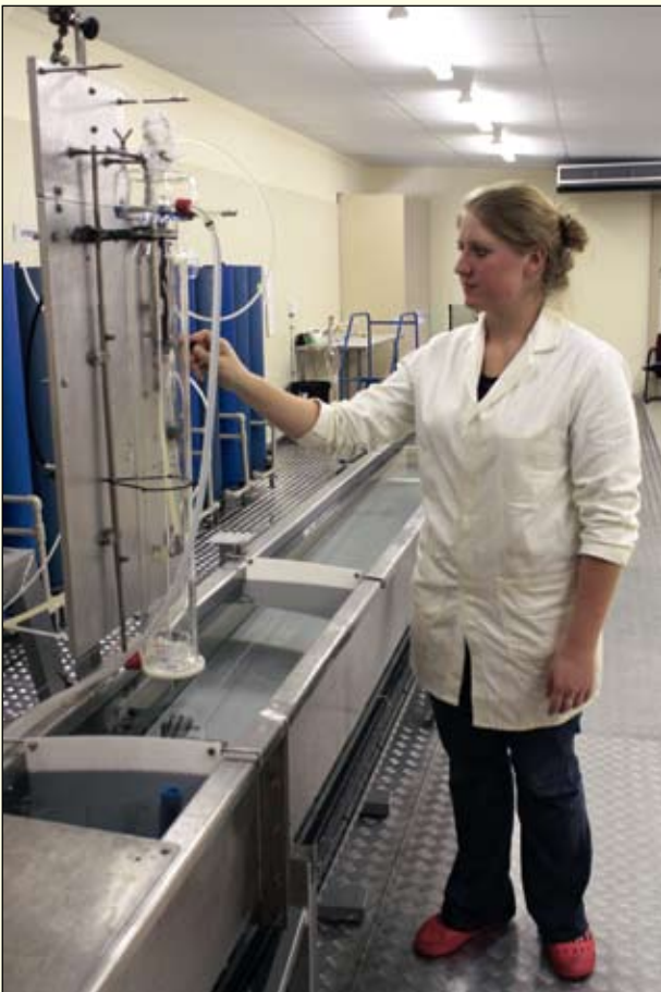
Ikusasa Water Plant Manager Anja Eysvogel inside the capillary ultrafiltration production facility.
