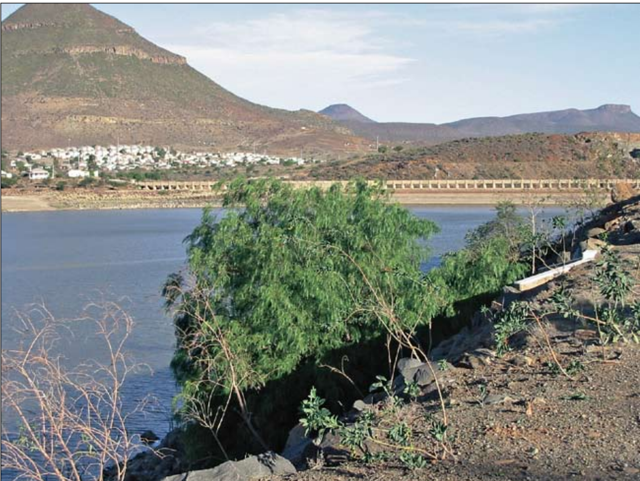
South Africa's Van Ryneveldspas Dam on the Sunday's River at Graaff Reinet has a catchment area of 12,382 km 2 . By 2009 it is estimated that there will be around 49,1 million m 3 of sediment in the reservoir, with a remaining storage capacity of only 29 million m 3 .
