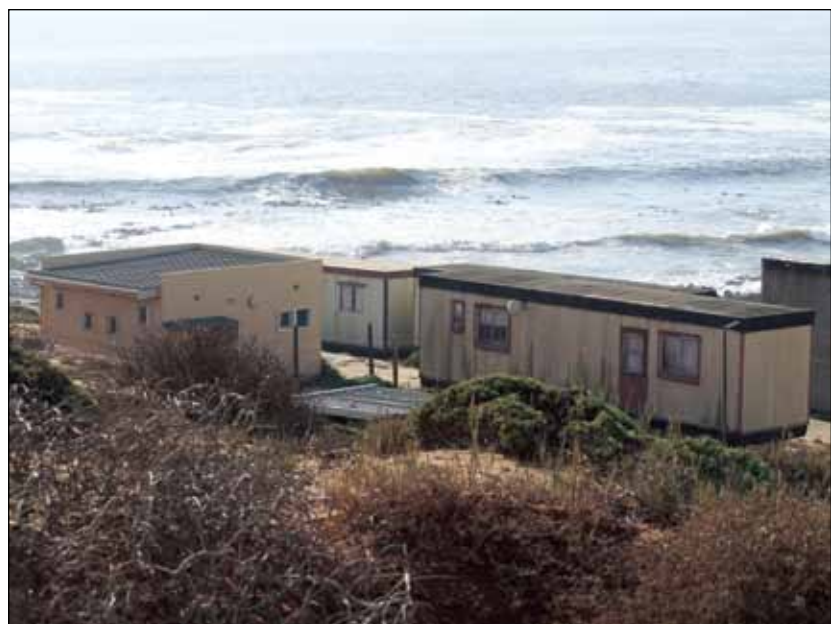
Mining accommodation at Namaqua Sands.
