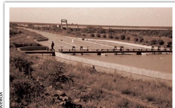
The Vaalharts weir and main canal in 1946. Three hand-operated radial sluice gates of 3 m by 2,7 m make up the inlet sluices. These flow into a three-barrelled aquaduct, which controls the water flowing into the canal.
