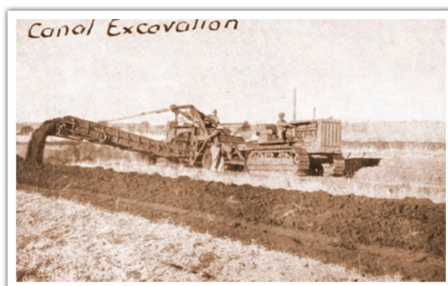
Bottom right: Mechanical and manual labour were employed at Vaalharts.
