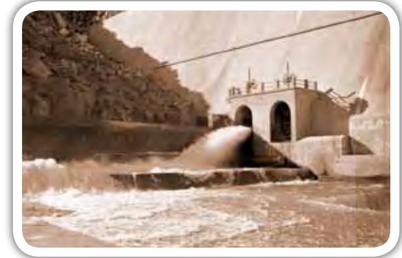
Top: The Clanwilliam Dam shortly after its completion. The original dam was a mass concrete gravity structure with a centrally situated overspill section.
