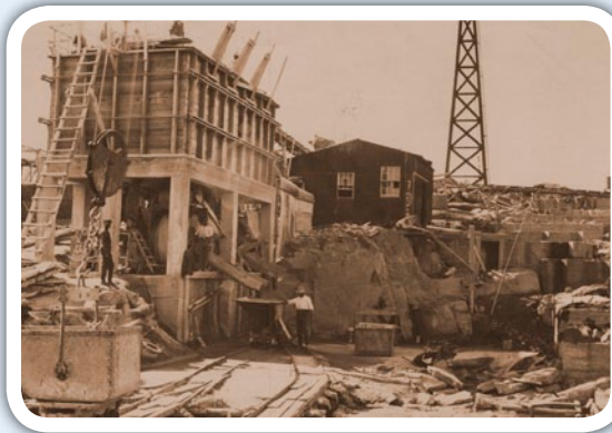
Left: Construction at the Kamanassie site progressed according to a strict programme set up by the Resident Engineer. Due to the inaccessibility of plant, mostly second-hand machinery was used.
