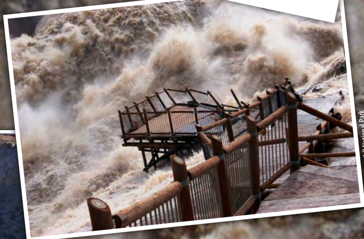
Above, middle and below: The wooden viewdeck at Augrabies snapped like a pack of twigs under the power of the Orange River.
