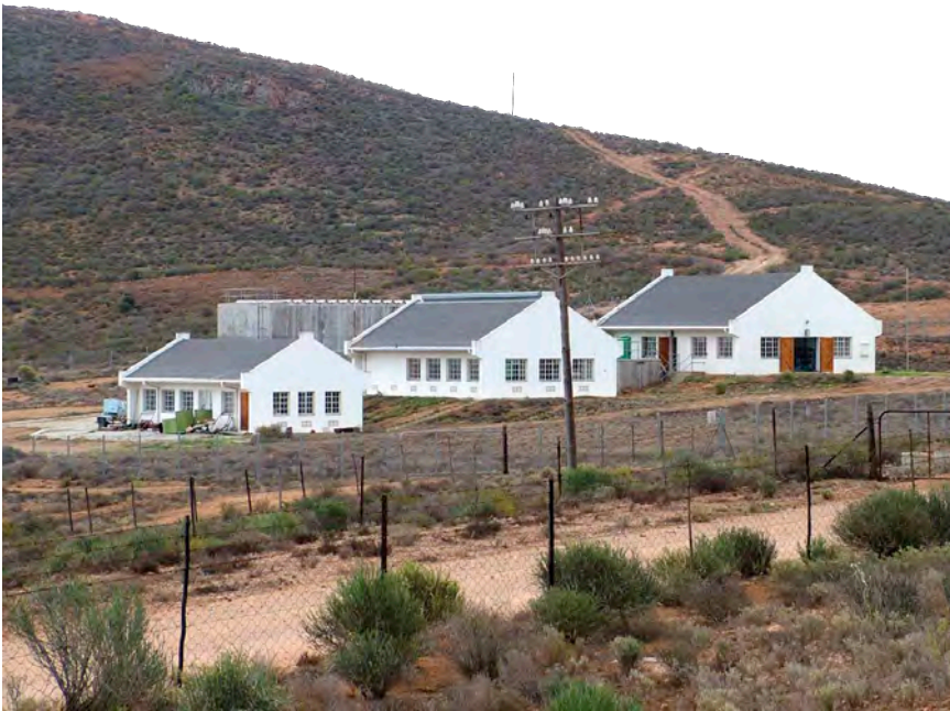
The desalination plant at Bitterfontein in the Western Cape was the first to be established in South Africa for domestic purposes.
