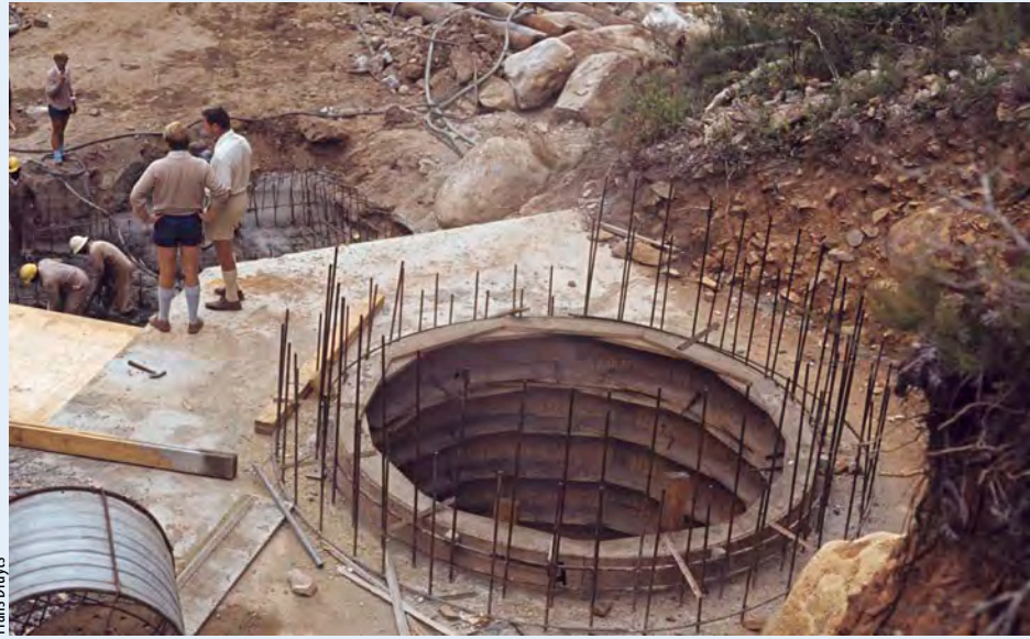
The Banhoek shaft under construction in 1979. The shaft is 162 m deep and 1,8 m in diameter.
