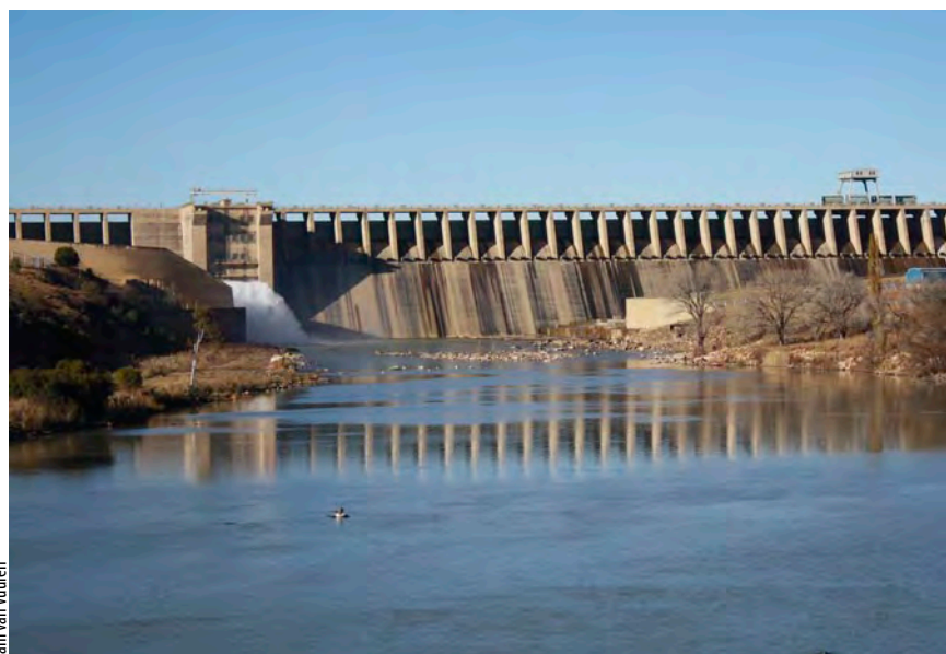
The Vaal Dam, constructed in the 1930s, remains the centre of Rand Water's supply infrastructure.
