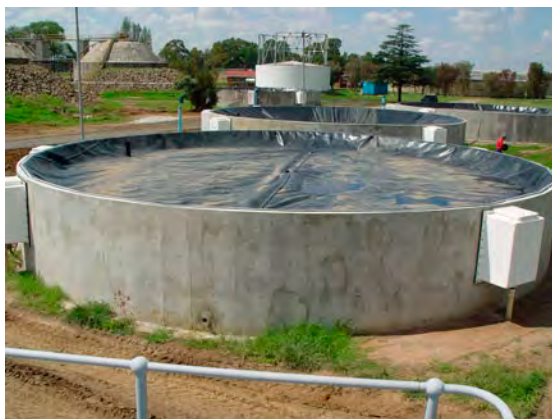
The establishment of the BioSure plant to treat acid mine-water using primary sewage sludge at ERWAT's Ancor works is a definite highlight in the WRC's history.
