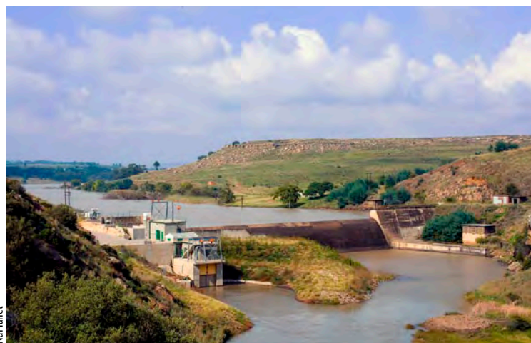
Bethlehem Hydro's 3 MW operation on the wall of the Sol Plaatje Dam.
