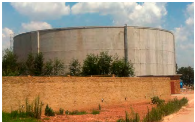
The Pierre van Ryneveld reservoir where the WRC-funded micro-hydropower solution has been installed.
