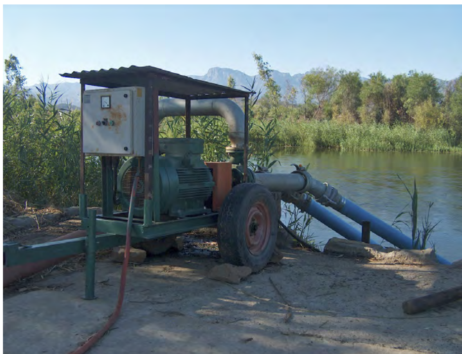
Irrigation water is sourced in a variety of ways, including direct river abstraction.
