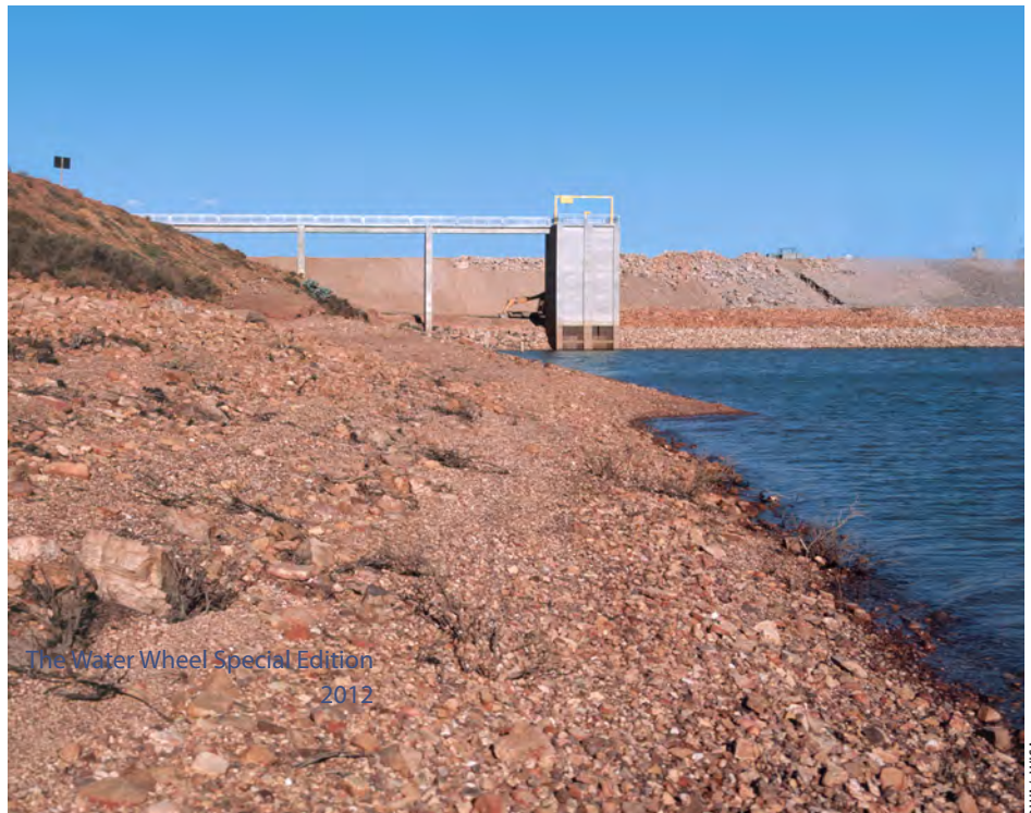
Above and left: In the 1980s the Greater Brandvlei Dam was created by the concurrent raising of the Brandvlei and adjacent Kwaggaskloof dams.
