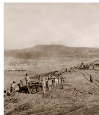
A view of the first Leeuw-Gamka Dam during construction in 1919 taken from the right bank.
