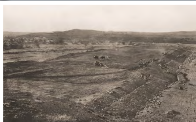
Dam from the left flank showing upstream slope and stone pitching in progress.
