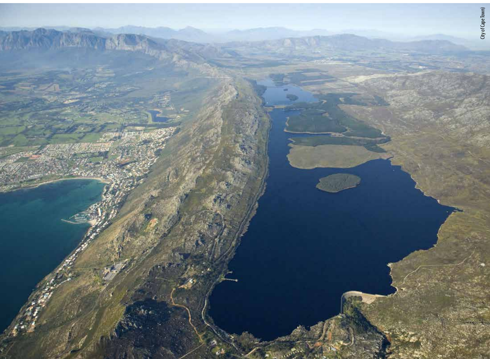
The two Steenbras dams as seen from the air.
