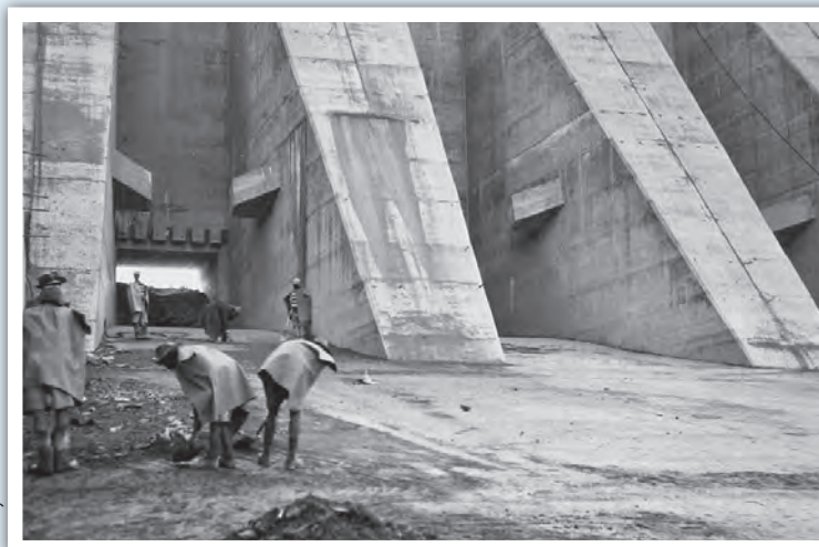
Construction of floodgates at Floriskraal Dam.
