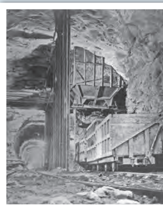
Left: The Orange Fish Tunnel during excavations.
