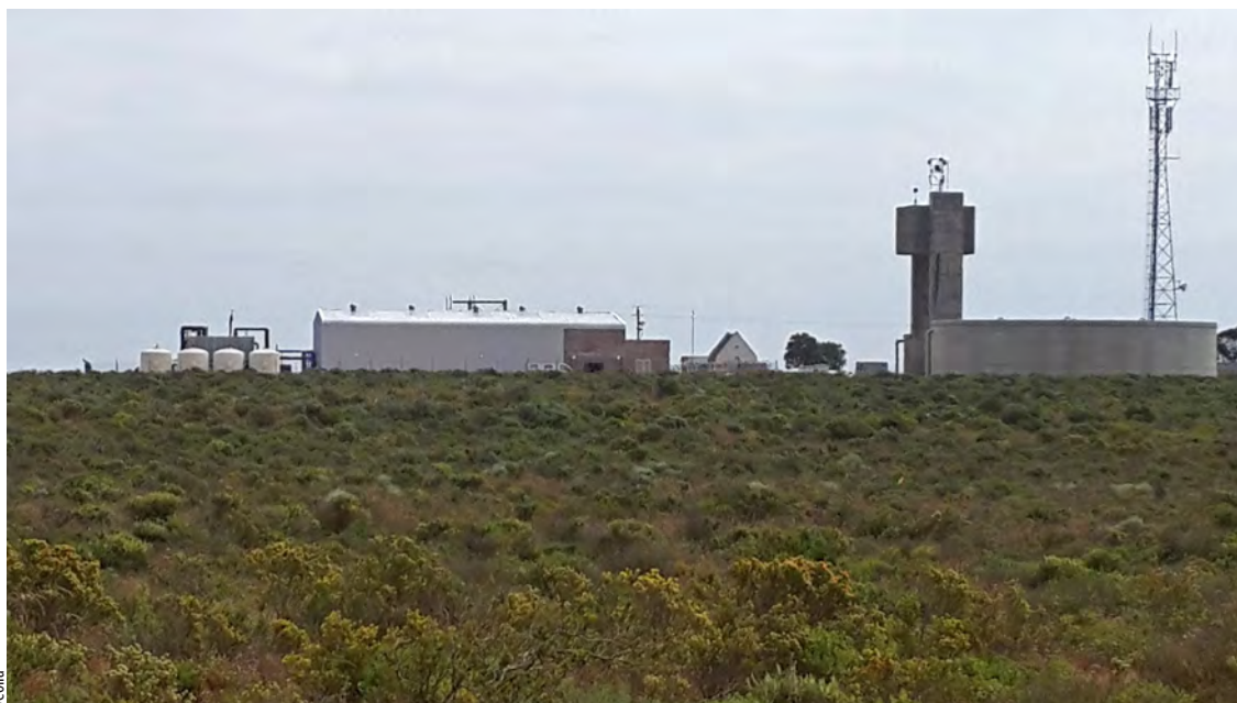
The new Lambert's Bay seawater desalination plant.
