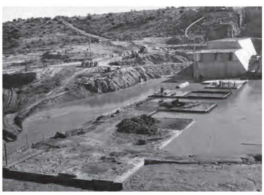
Top: Leeuw Gamka Dam nearing completion.
