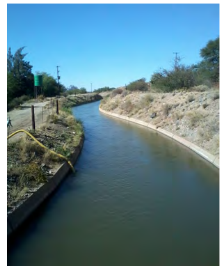
Below: A typical irrigation water canal.
