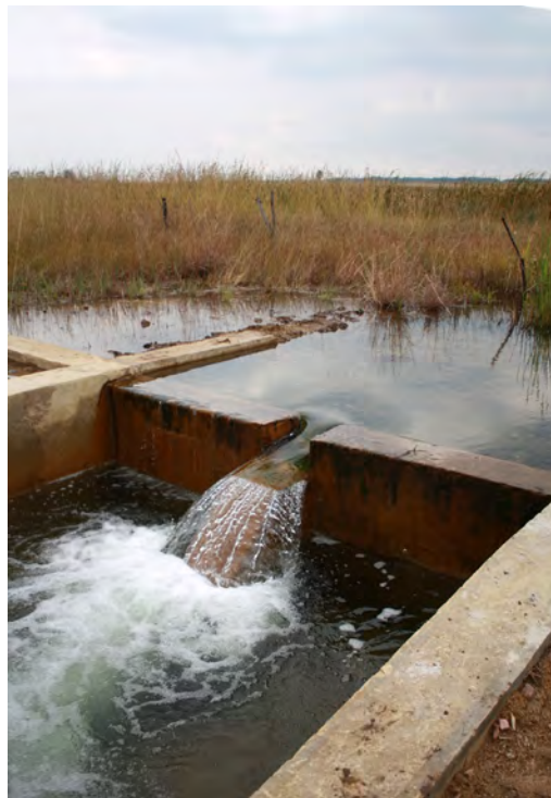
One of the concrete structures constructed in the wetland.
