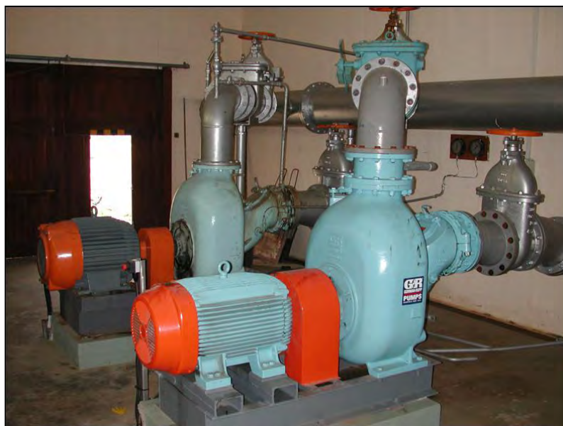
Figure 5.19: Typical dry-well installation (above ground level)
