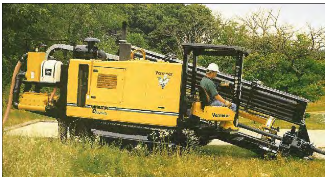
Figure 3.19: Directional drilling and installing of small-bore sewer
