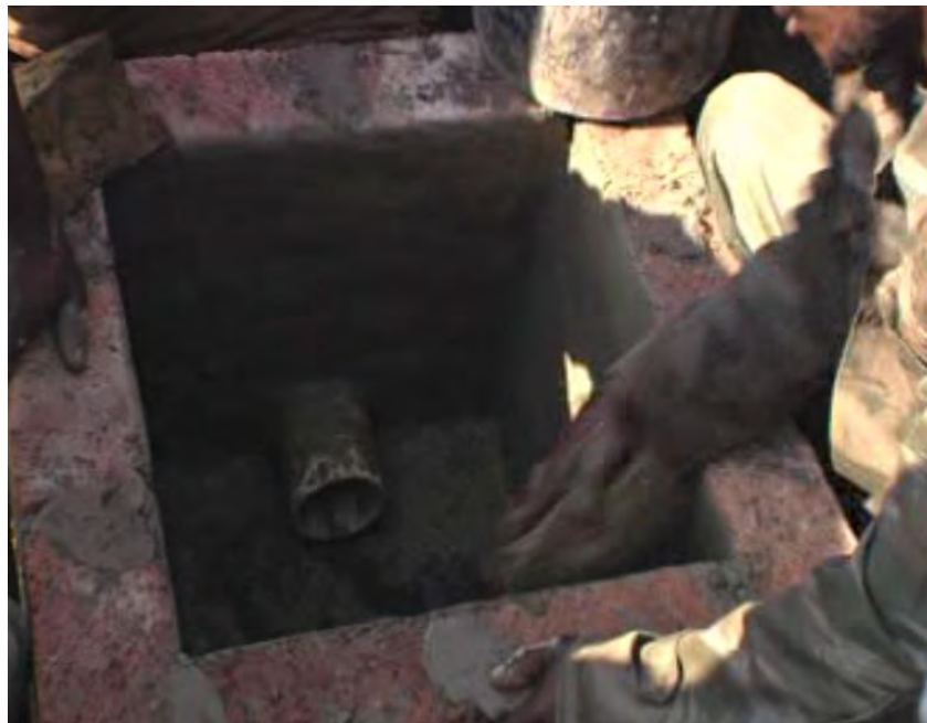
Figure 8.2: Construction of inspection chamber (Eslick and Harrison, 2004a)
