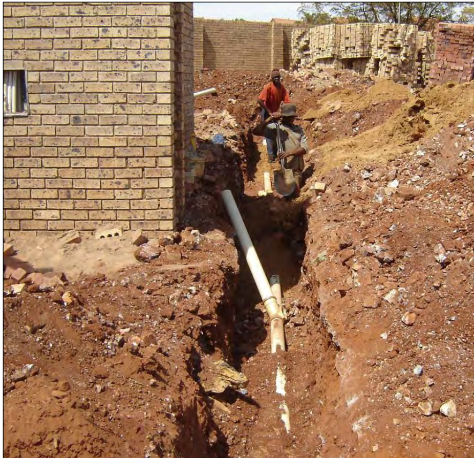
Figure 3.6: Construction of on-site sewer connection (conventional gravity sewer)
