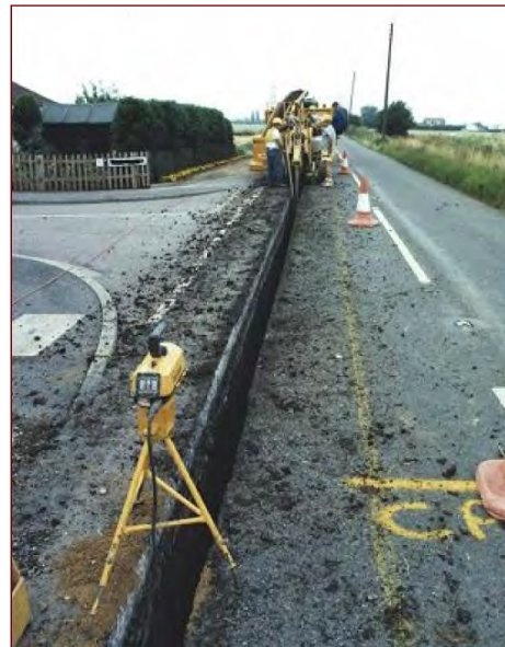
Figure 3.13: Excavating trenches (QUA-VAC, 2009)
