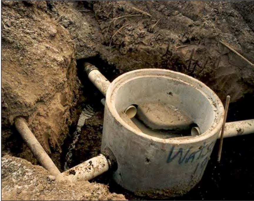
Figure 3.5: Typical manhole with benching (circular)
