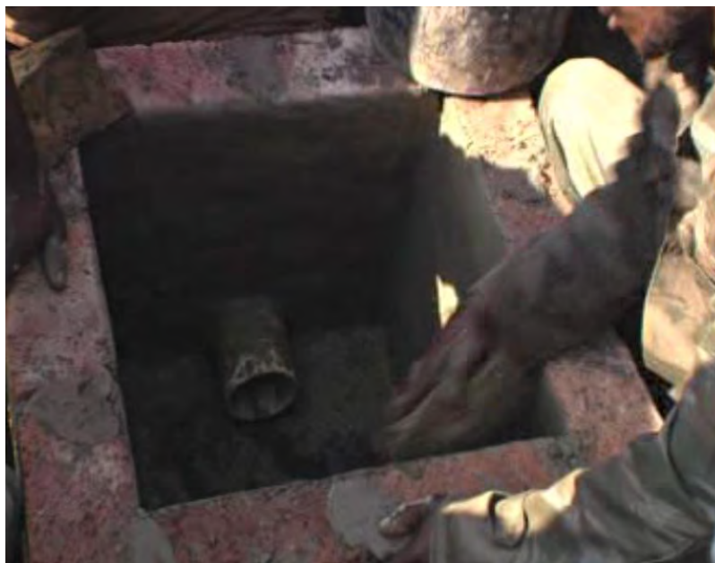
Figure 3.24: Construction of inspection chambers (Eslick and Harrison, 2004a)
