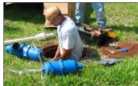
Figure 3.14: Contractor installing vacuum valve in valve pit
