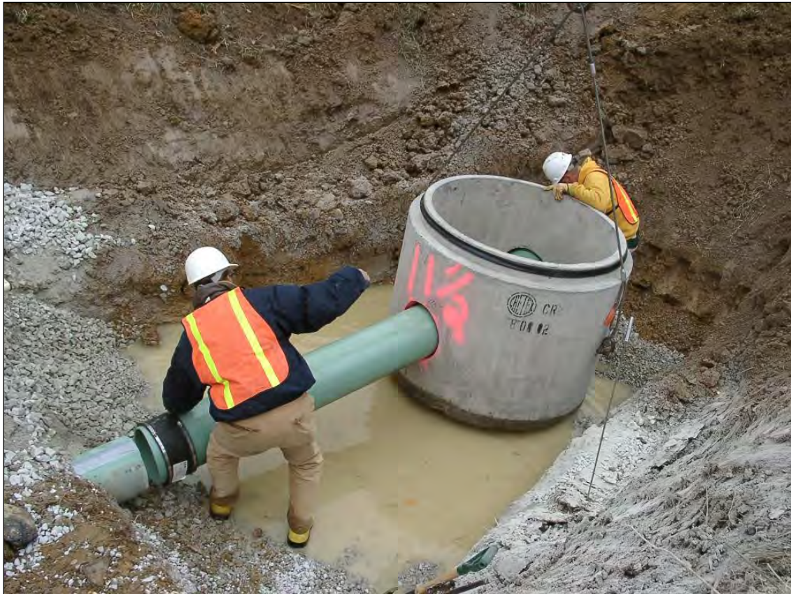
Figure 3.7: Construction of connector service (conventional gravity sewer)
