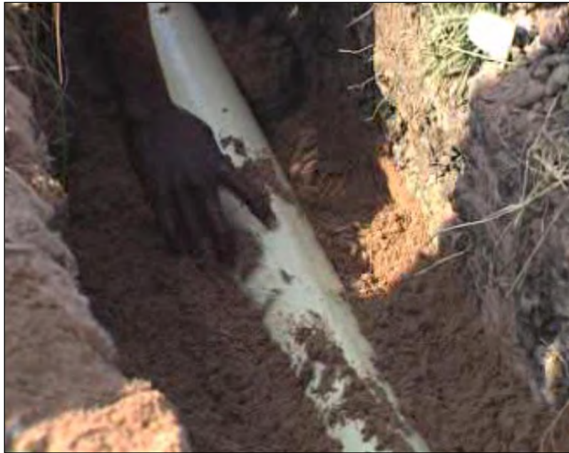
Figure 3.23: Installing the shallow sewer (Eslick and Harrison, 2004a)
