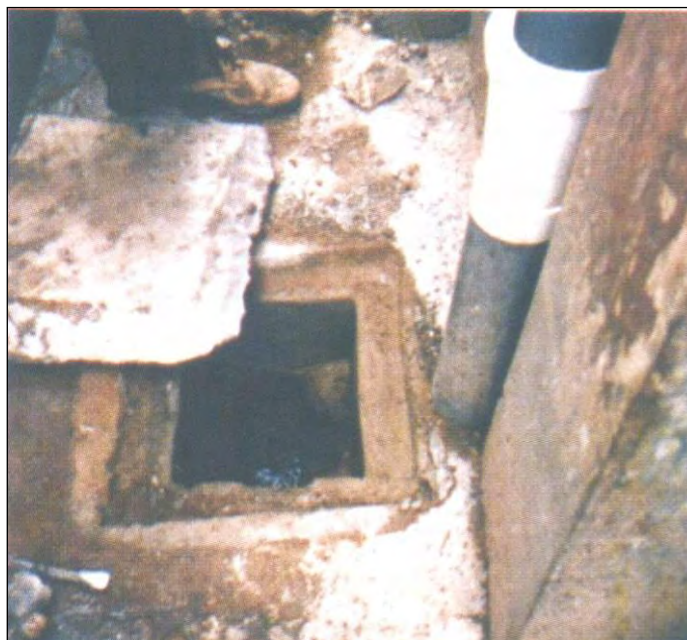
Figure 3.21: Household inspection chamber (Pegram and Palmer, 1999)
