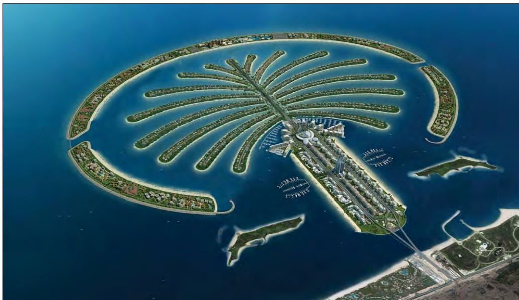
Figure 3.10: Palm Jumeirah in Dubai utilizes a vacuum sewer system
