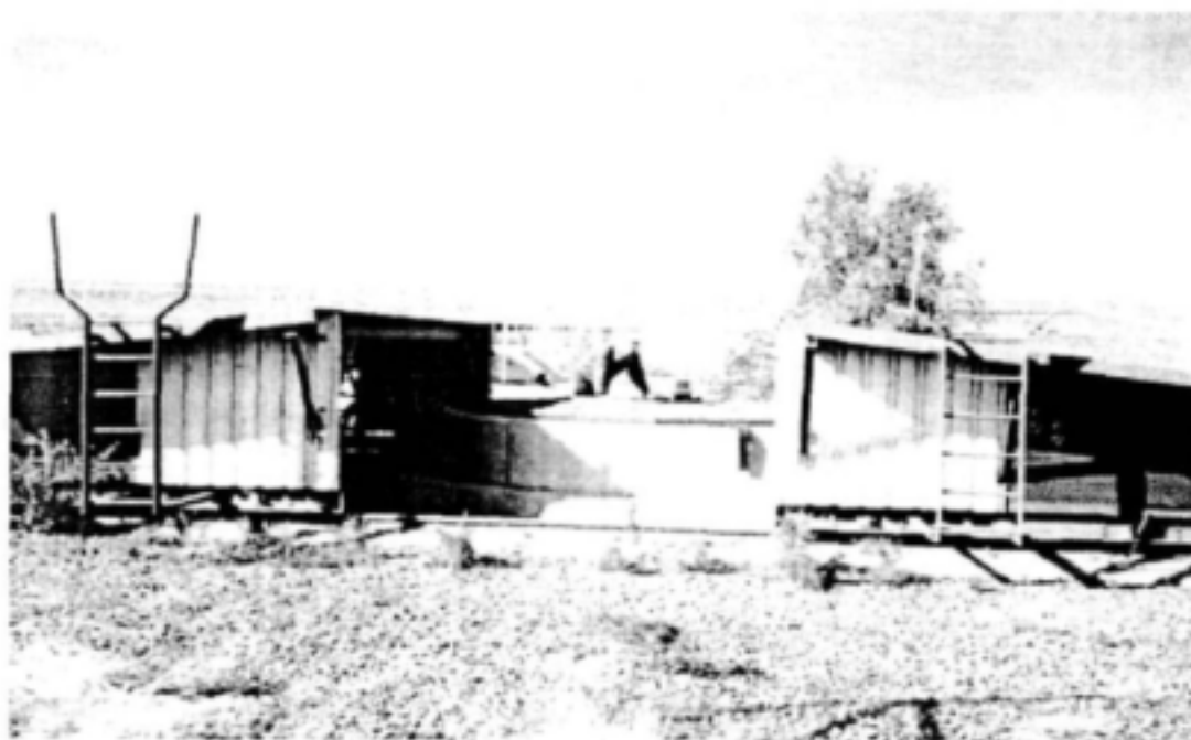
Figure 8.1.2-9 Depth recording at Orange-Fish Tunnel shaft.
