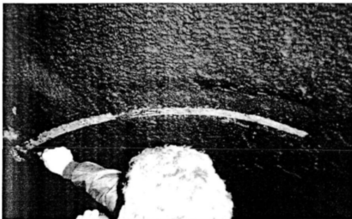
Figure 5.8.6-2 Sediment deposition in Roode Elsberg Tunnel
