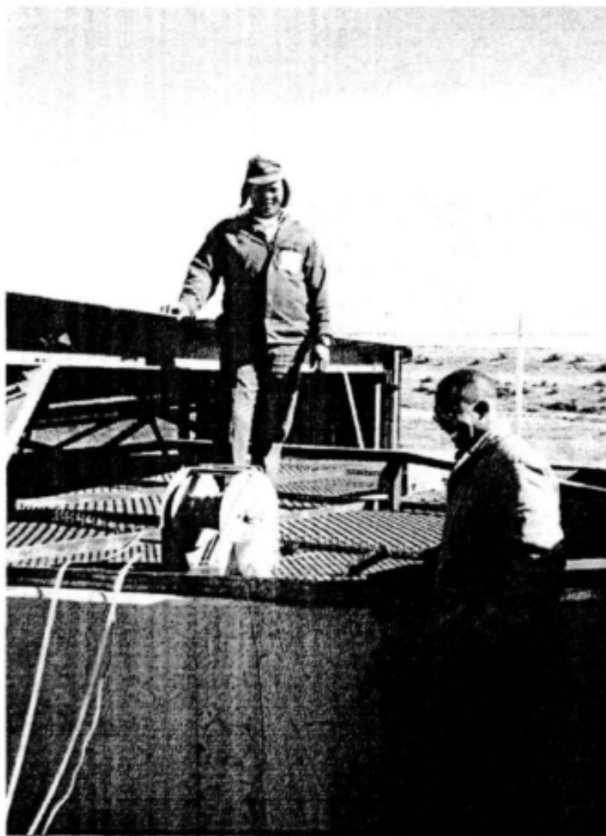
Figure 8.1.2-8 Depth gauge at tunnel shaft operated by DWAF personnel
