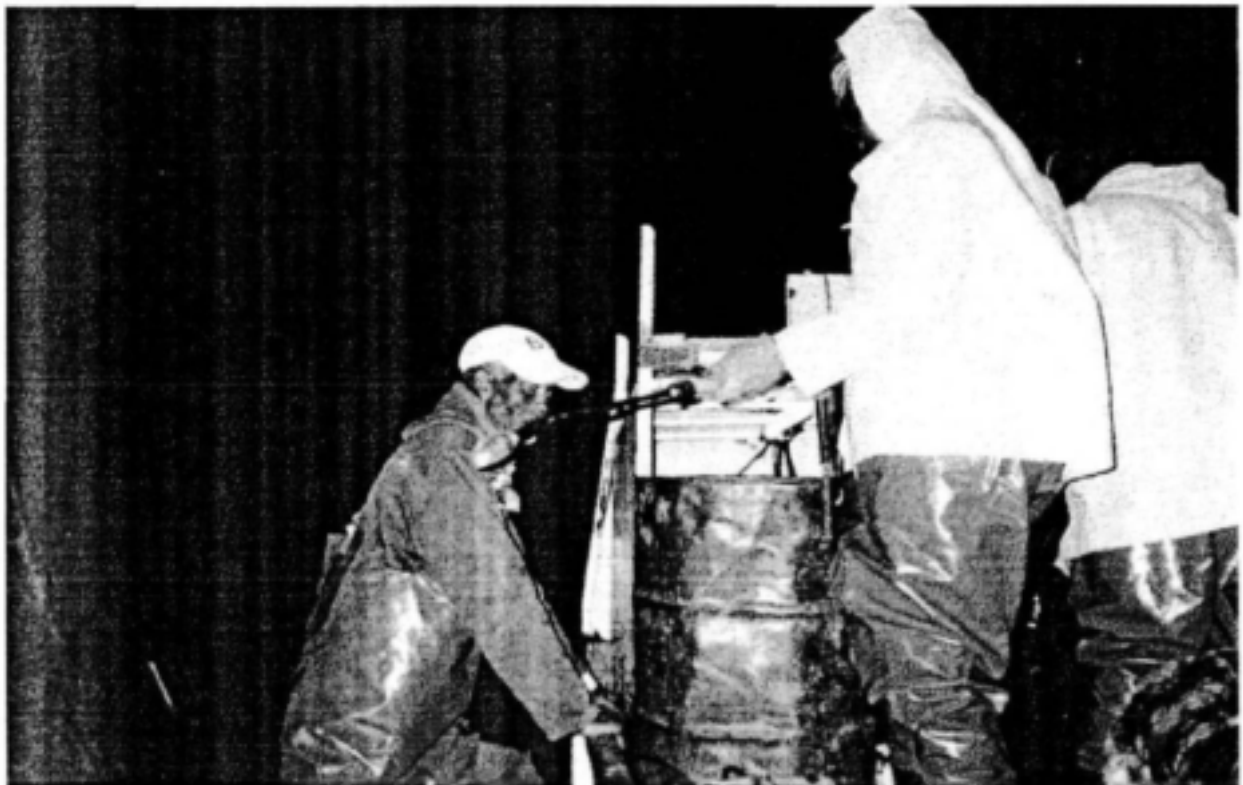
Figure 8.2.5-2 Cleaning team on truck in Orange-Fish Tunnel
