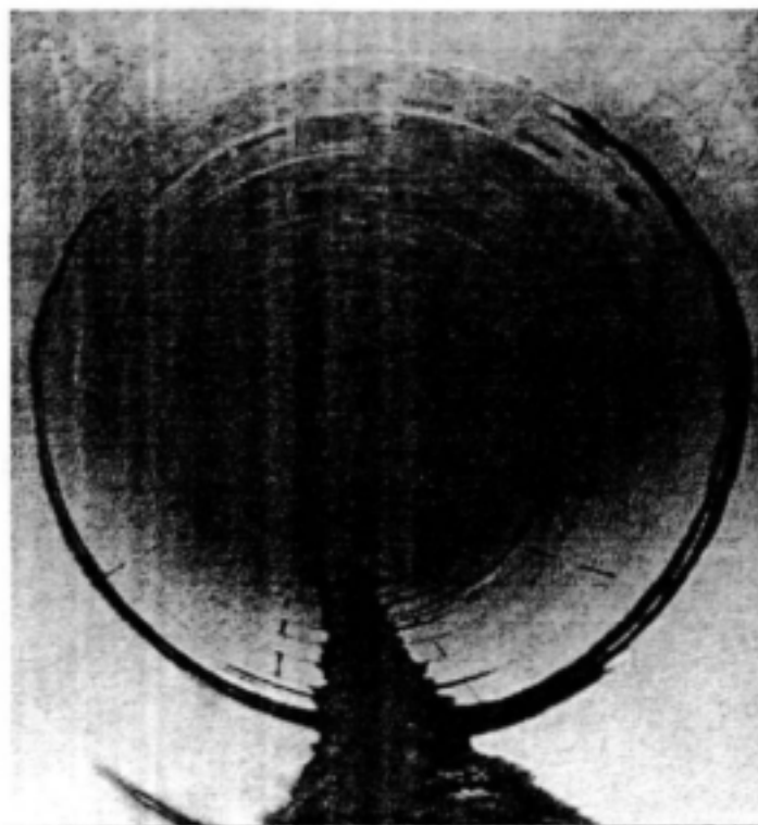
Figure 5.3.3-1 Segmentally lined Delivery Tunnel North
