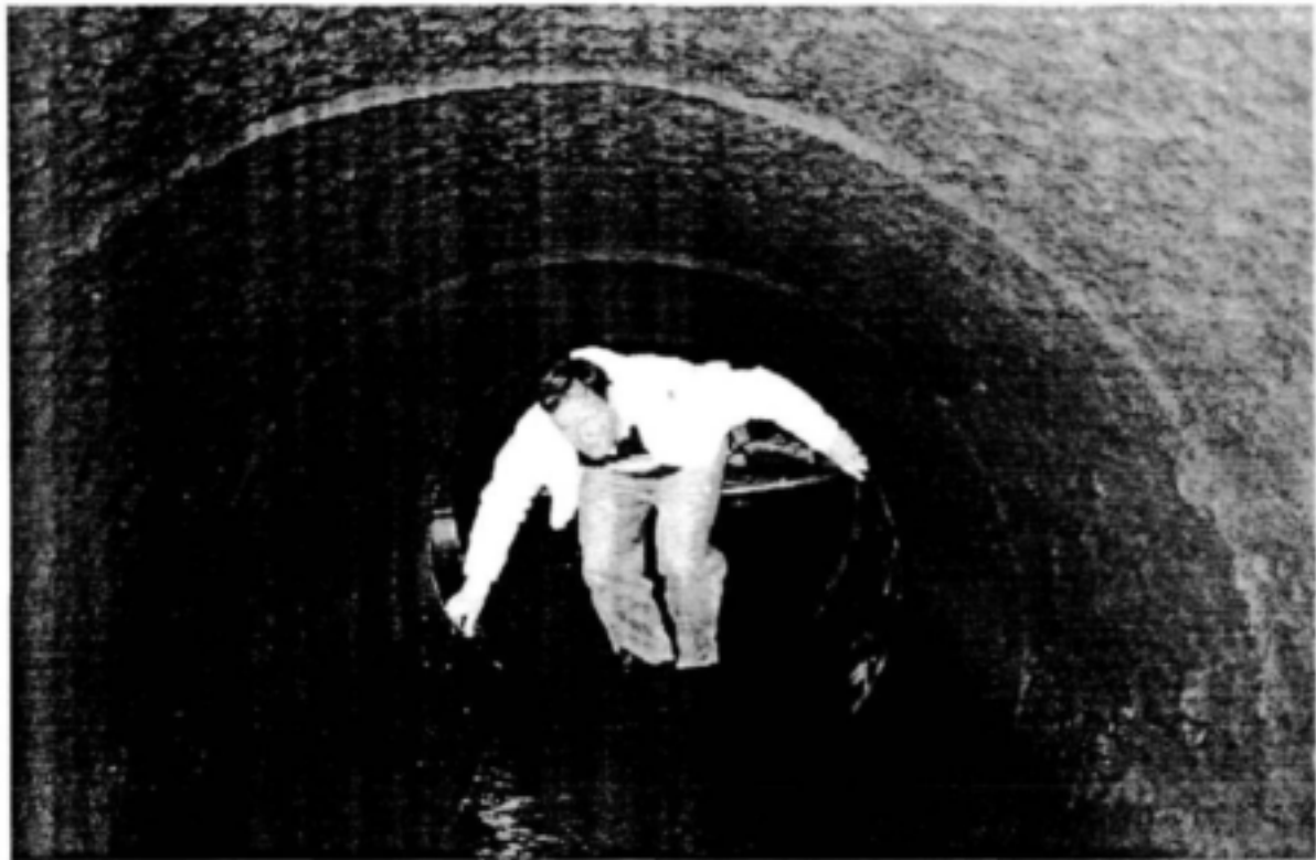
Figure 8.1.4-4 Roode Elsberg Tunnel at intake
