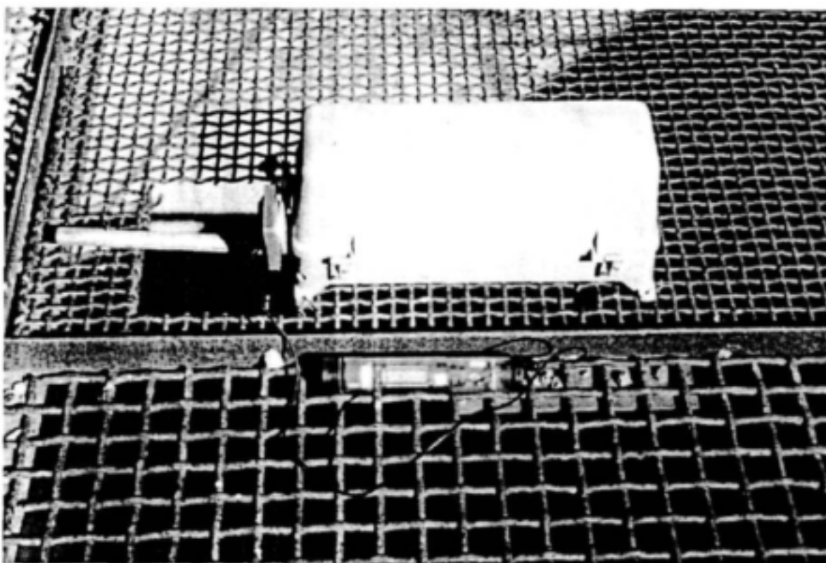
Figure 8.1.2-10 Ott water level reader and Thalimedes data logger
