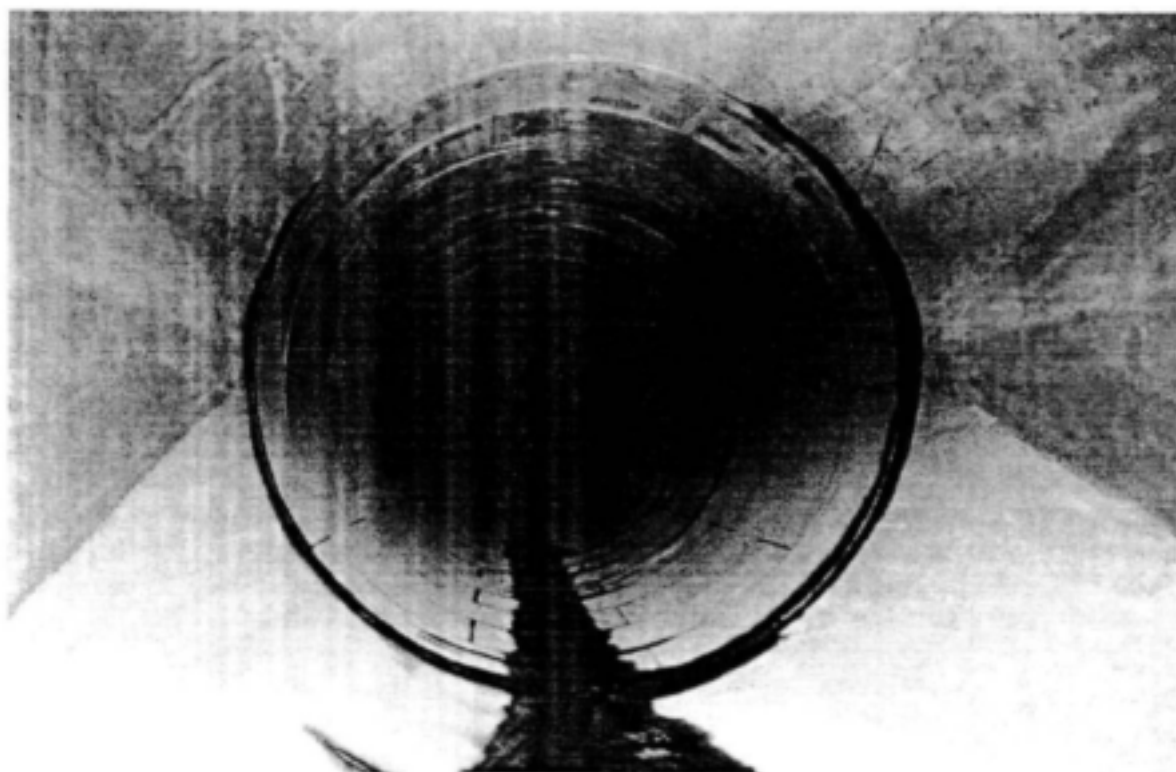
Figure 9.1-5 Delivery Tunnel North at Ash River
