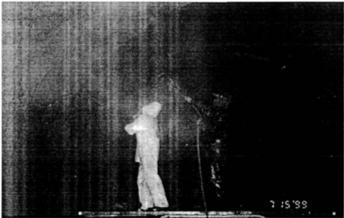
Figure 8.2.6-1 Theewaterskloof Tunnel cleaning during 1999
